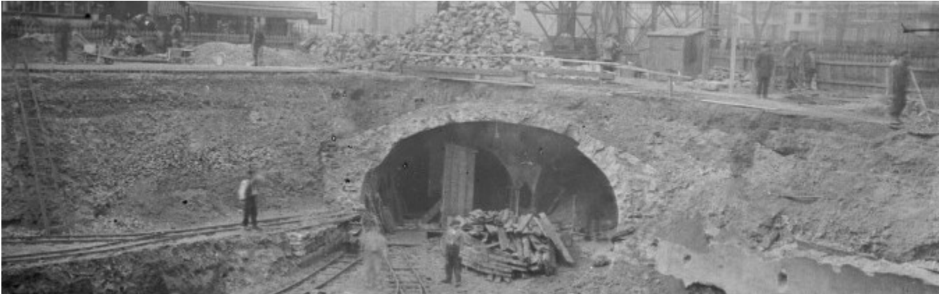
Figure 1: Construction of the Paris Metro in 1902-1910.
